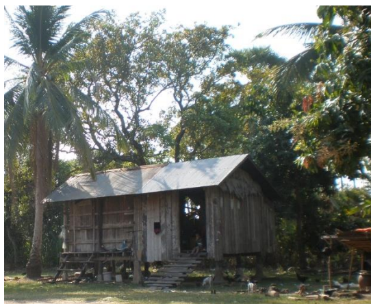
Cambodian home showing signs of improvements such as timber walls, metal roof and an extension to its size. (photo QSA)
